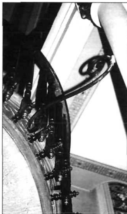
Figure 2. Iron support bracket (unmentioned in published accounts) reveals the "miracle" is a partial one. (Photos by Joe Nickell)
